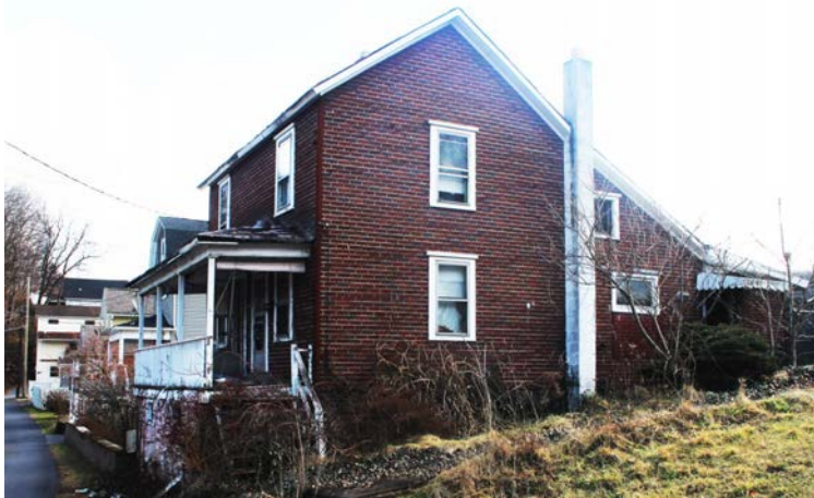
At near left is a home at 70 Ridge Street, formerly associated with the Gamulka and Kotch Families. Thomas William was later owner. Additional properties are being evaluated for demolition in the near future.
